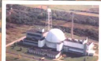
SPACE POWER FACILITY
